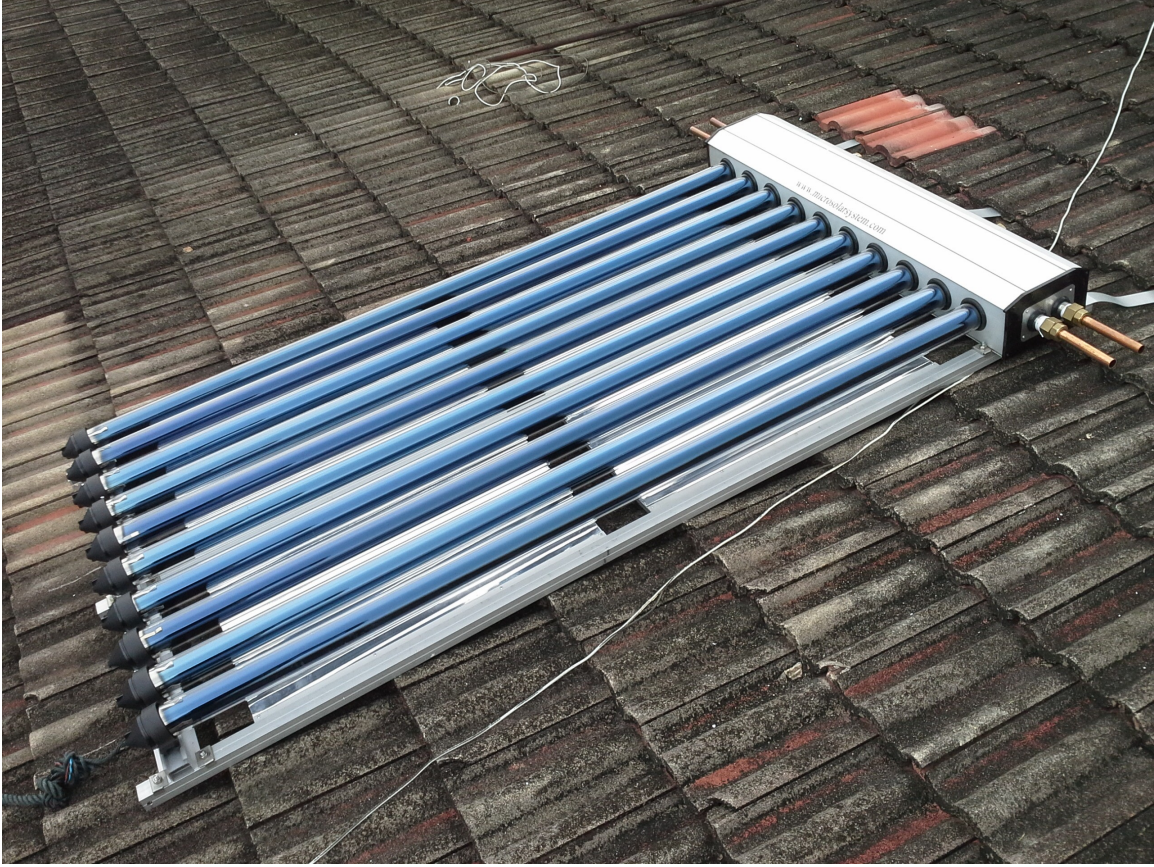
20130322 Microsolar Manifold used for Solar Hybrid Air Conditioning
