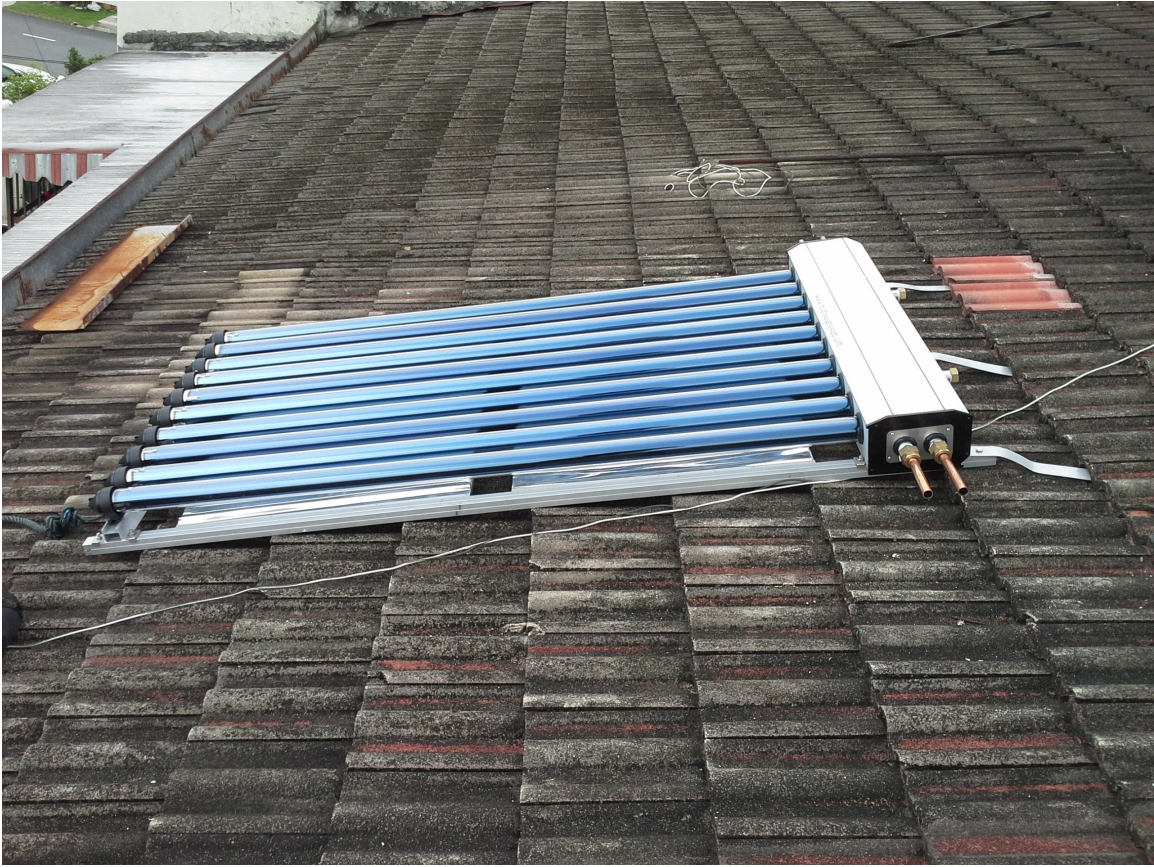
20130313 Microsolar 10 tubes Manifold Model being installed for Solar Air conditioning at Solar Dingin's Showhouse in Ampang Jaya , Kuala Lumpur , Malaysia.
