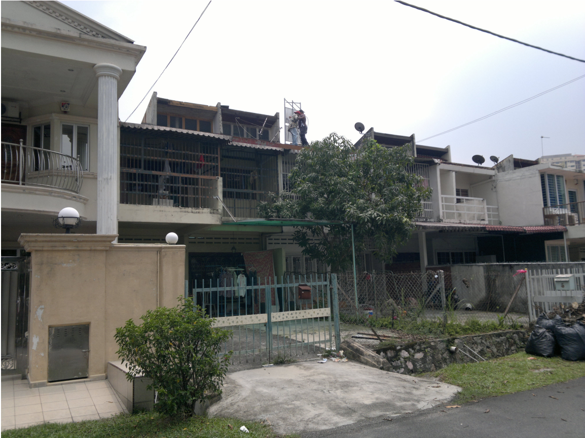
20130313 Installing the frame of Microsolar Manifold for Solar Air conditioner on roof at Ampang Jaya , Kuala Lumpur, Malaysia.
