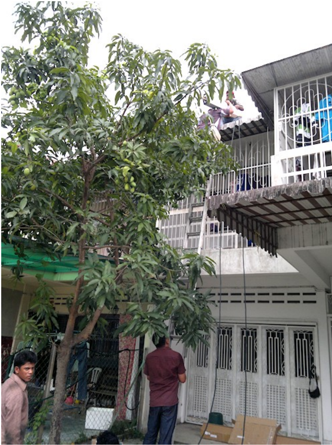
20130313 Installer Kevin Lim carrying the Microsolar Manifold model up onto the roof to be installed as a solar hybrid air conditioner at Ampang Jaya , Kuala Lumpur , Malaysia for our partners Solar Dingin Sdn Bhd.
