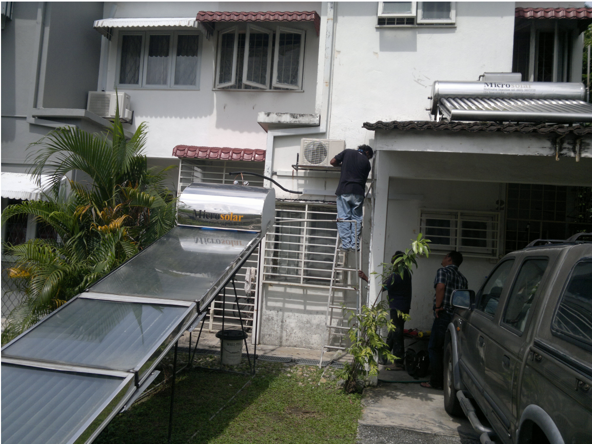
20130107 The original 1999 vintage Microsolar Nepal Prototype Model being converted to be used as a solar air conditioner and connected to the air conditioning compressor at Microsolar's showhouse in Subang Jaya Selangor Malaysia. The current Microsolar Water Heater Vacuum Tube model can be seen on the car porch roof at top right. The Microsolar Hybrid Solar Air Conditioner provides a 38% savings on electricity usage when used as a solar air conditioner.
